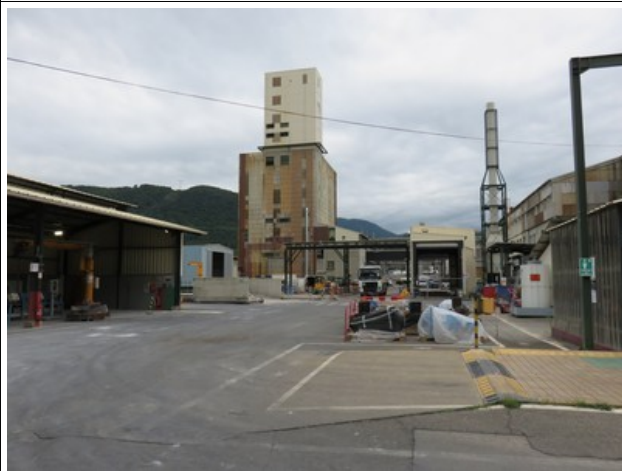
Rack Sud+ bassins tampon
